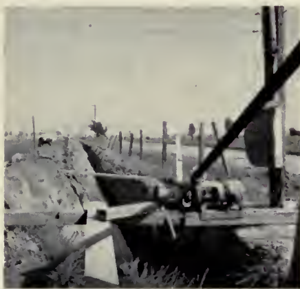
FROM DRAIN TO MAIN DITCH. —At immediate right, water is pumped to the main ditch. At far right, the main ditch, with water that is going to be used over again.
